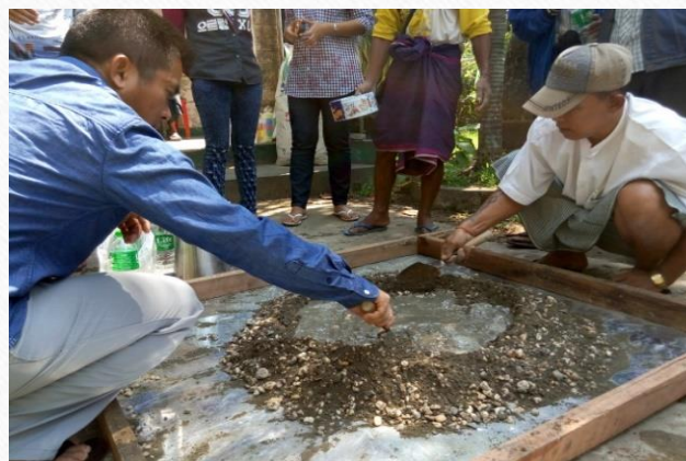
Safer Construction (concrete), by Myanmar Engineering Society
