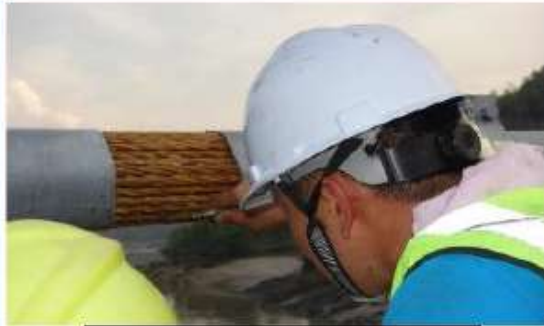
Main Cable Inspection
