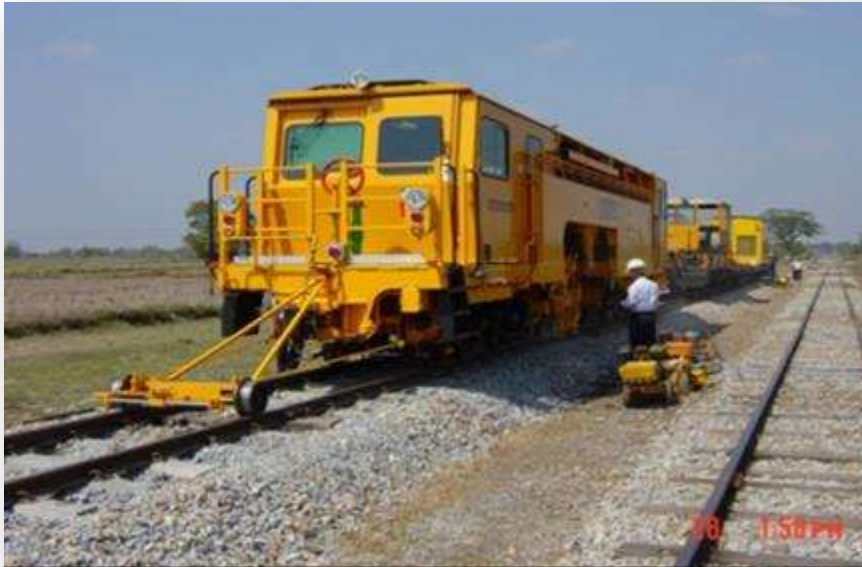
Track Maintenance with Automatic Leveling, Lining and Tamping Machine
