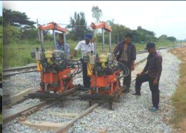
Ballast Tamping with Hydraulic Off Track Tamping Machine
