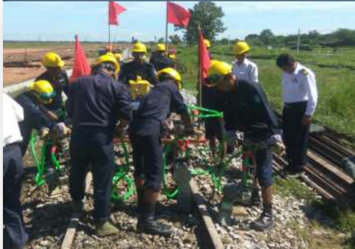
Ballast Tamping with Hydraulic Off Track Tamping Machine
