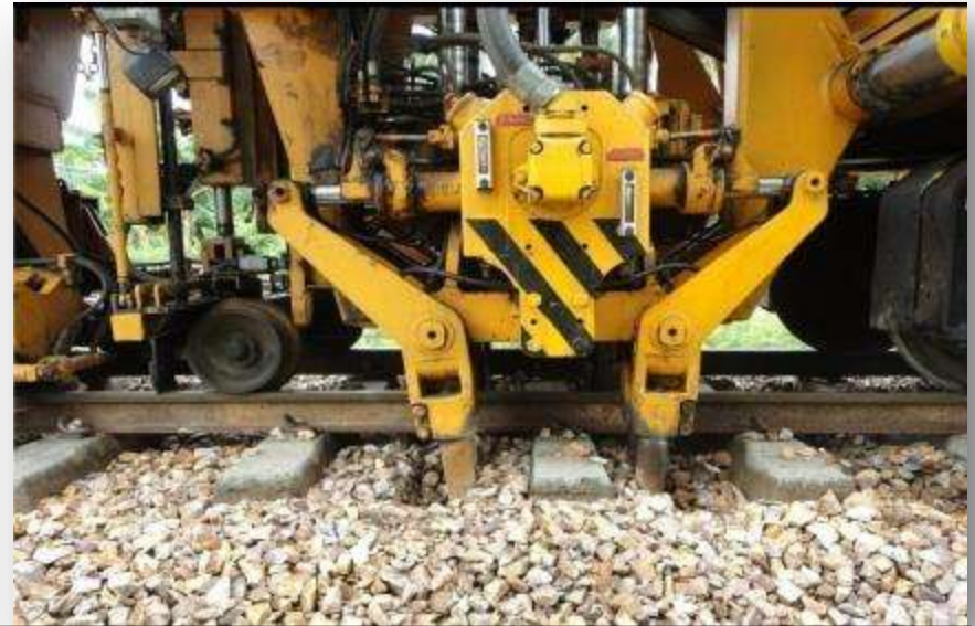
Track Maintenance with Automatic Leveling, Lining and Tamping Machine
