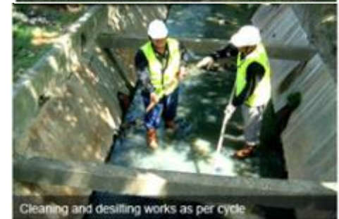
Cleaning and desilting works as per cycle
