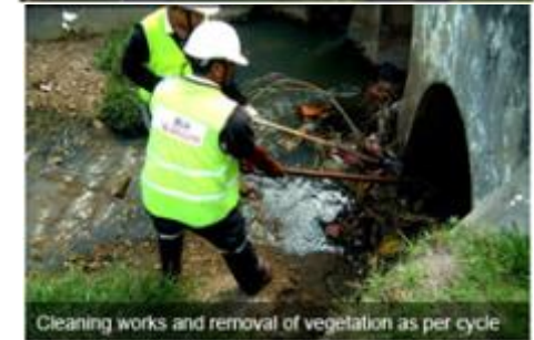
Cleaning works and removal of vegetation as per cycle
