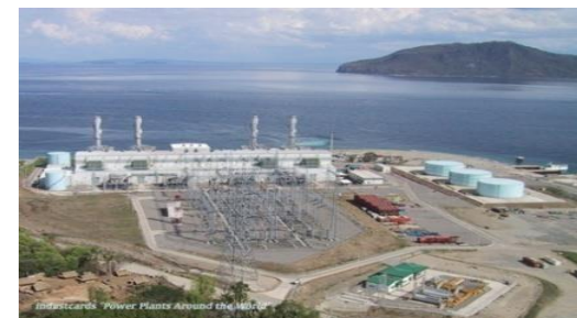
1,200 MW Ilijan Power Plant NPC IPP(KEPCO)
