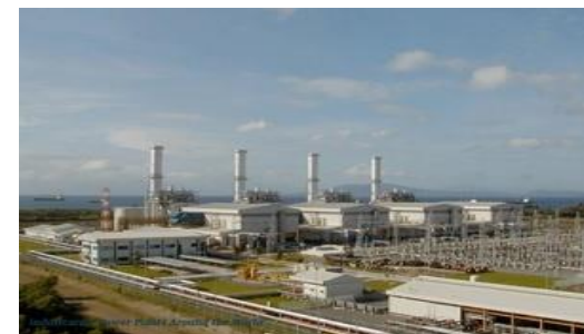
1,000 MW Sta. Rita First Gen/ IPP
